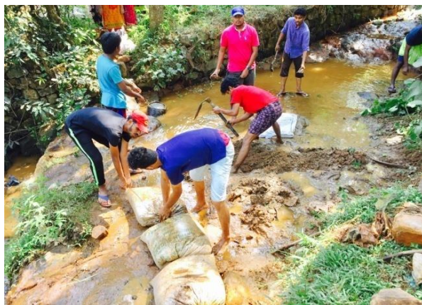
Check Dam Construction
